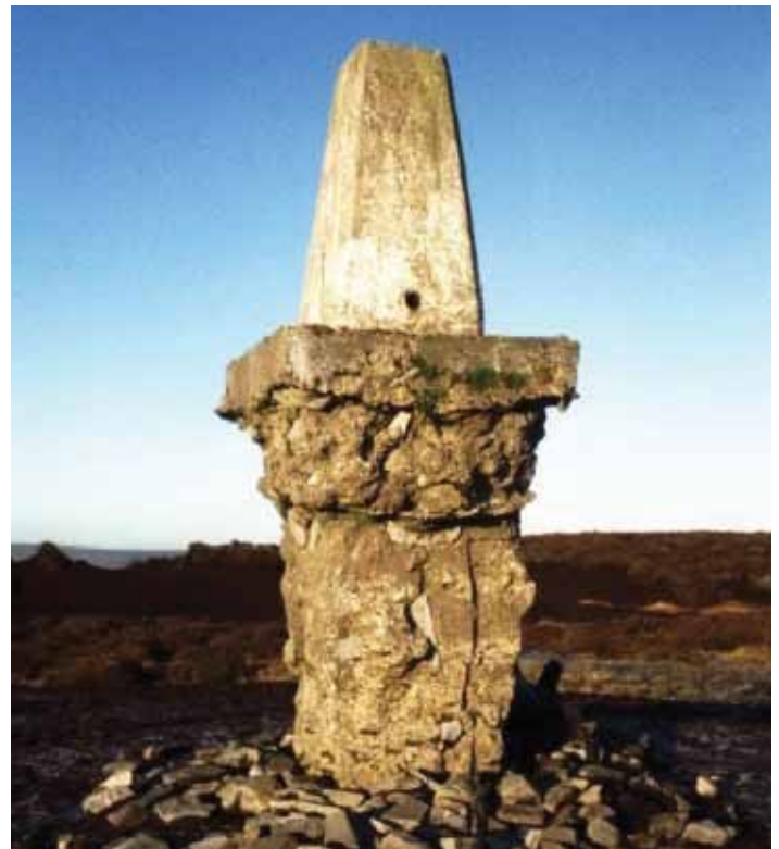
Trig point built on boggy soil, now eroded, showing the large fraction of the pillar that lies underground
