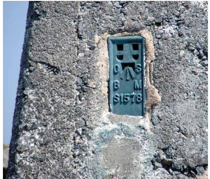
On one side there is an indentation with a metal plate and here is found the benchmark
